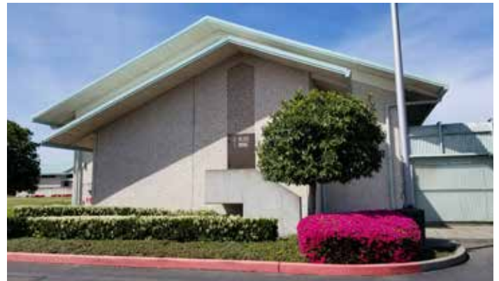
Remann Hall - Dorm Entrance from parking lot
